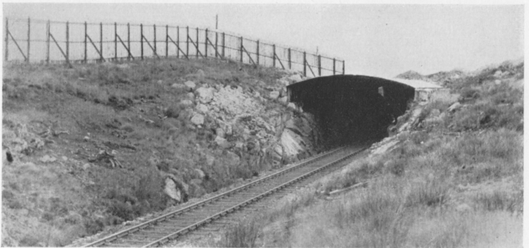
Snowshed in Cruach rock cutting. South end (top), Interior (centre), North end (bottom)
